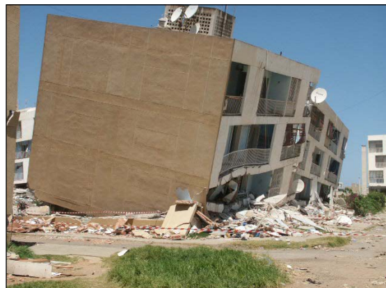
Figure 28 Total disappearance of the first floor.
