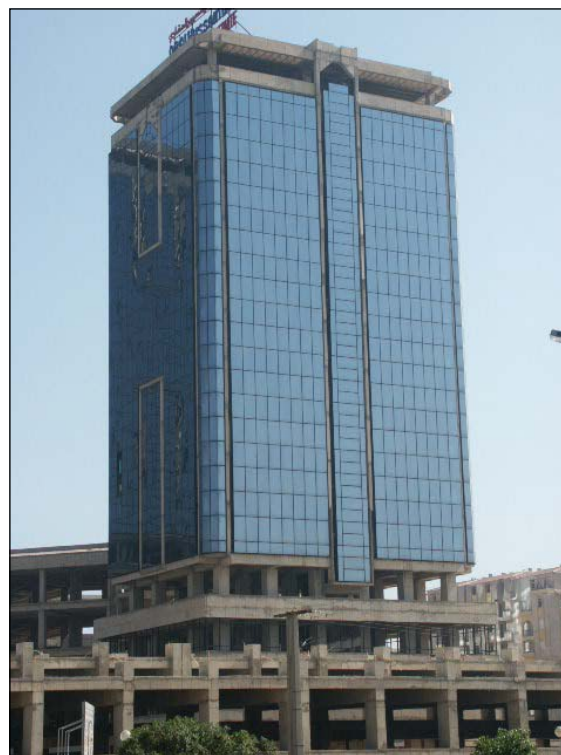
Figure 36 No failure of the glazing system of an R/C high-rise building.
