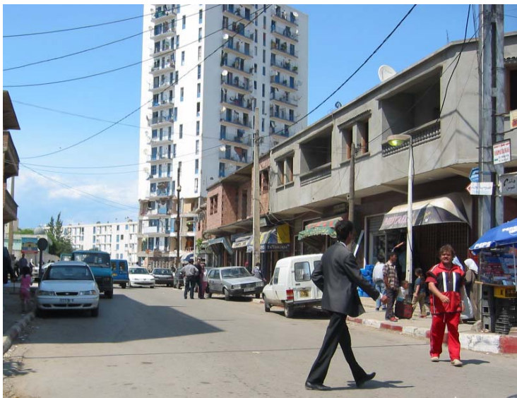
Figure 57 Apartment tower in Reghaia heavily damaged in the main shock. This photo shows an evacuated tower three hours before its total collapse during the first strong aftershock (M5.8).
