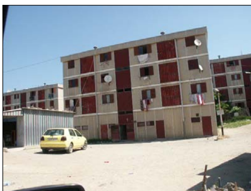
Figure 35 No failure of steel-frame structure with lightweight infill panels.
