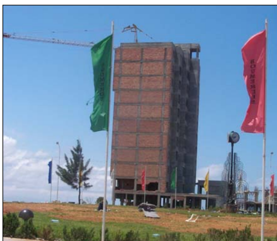
Figure 37 11-story RC frame building in Boumerdes — no damage in resistant structure.
