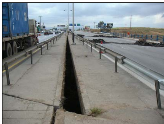
Figures 46 a and b Damage to Highway 5 Bridge.
