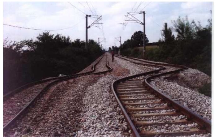
Figure 30: Railroad track distorted by an earthquake. A 2.3 m co-seismic displacement has distorted the railroad track near the railway station Tepetarla in the region between Sapanca Lake and Izmir Gulf. Taken from http://www.geo.tudelft.nl/fmr/research/insar/izmir/railroad.jpg .
